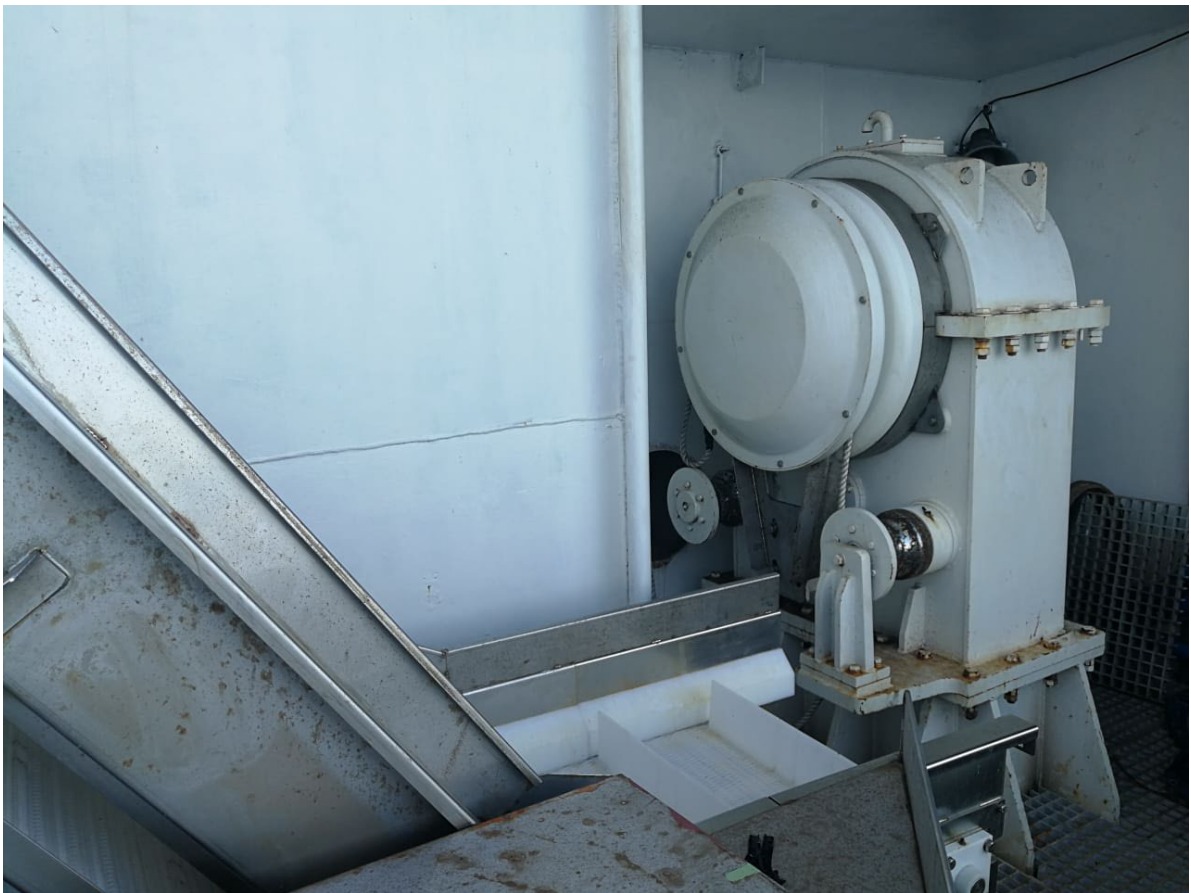
Figure 6: Hydraulic winch and transporter
